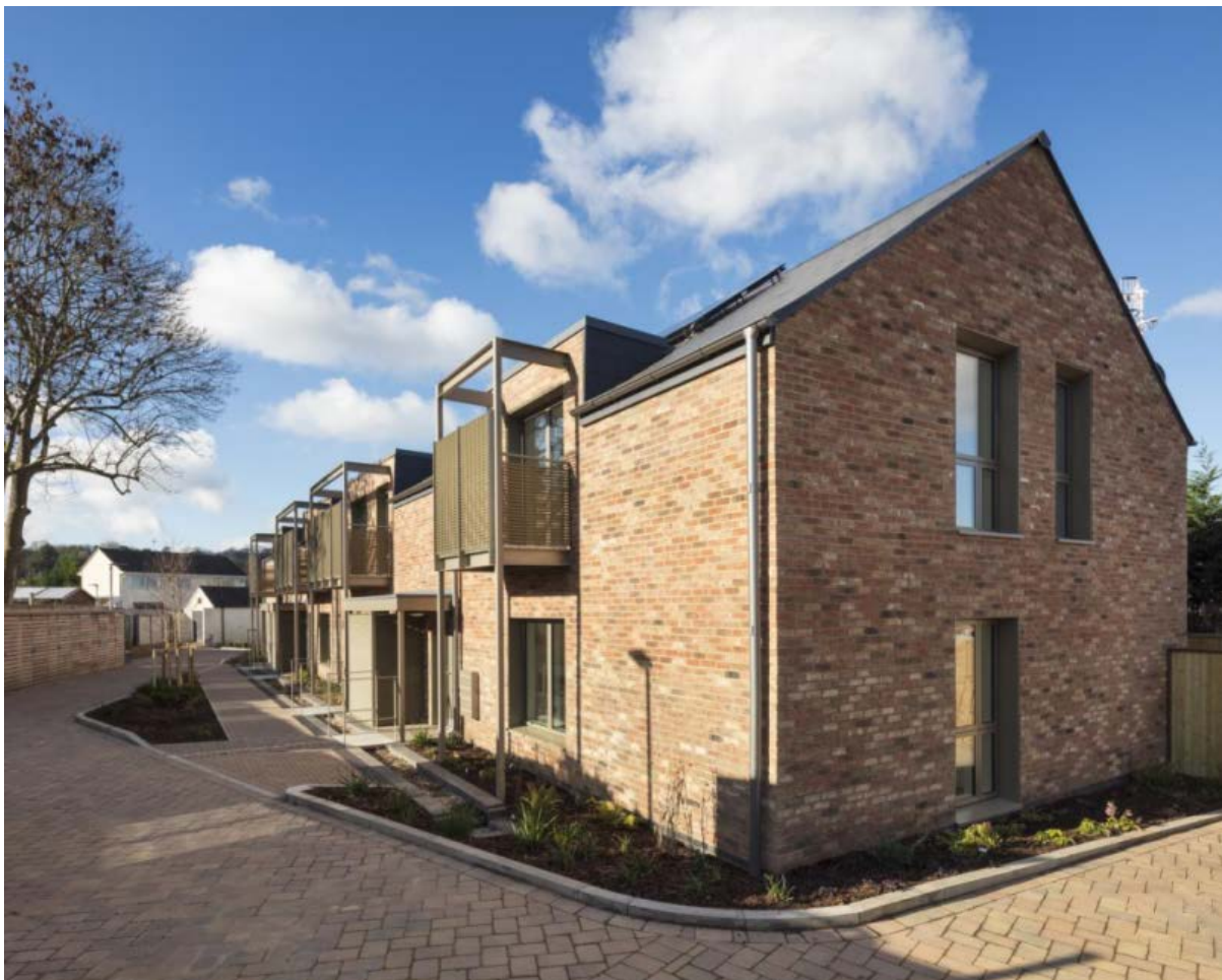
Award winning new council homes at Henbury
